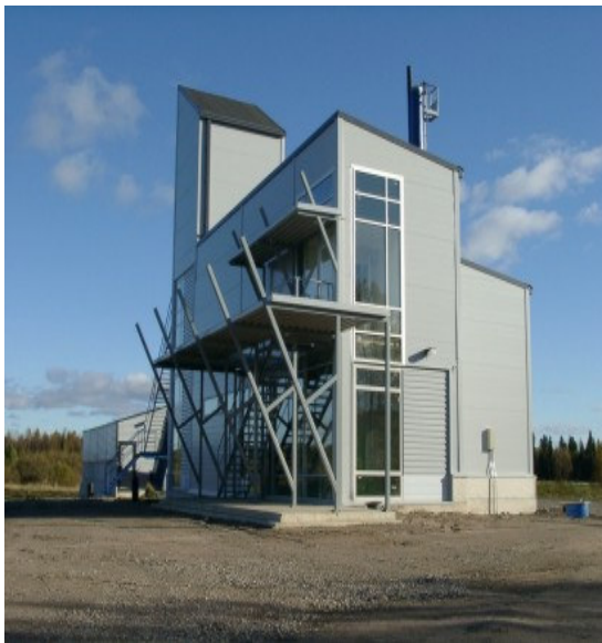
Figure 1. Entimos power plant in Tervola, Northern Finland
