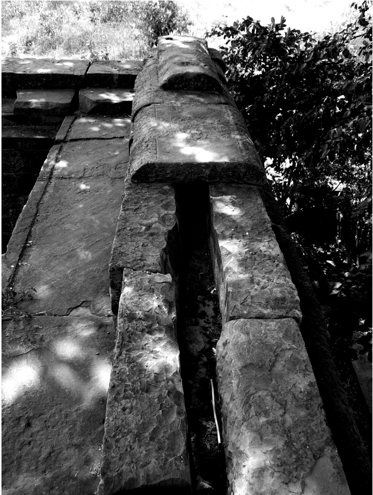
6. Behṛi Math (District Ashoknagar, MP). Roof parapet with cap stone.
