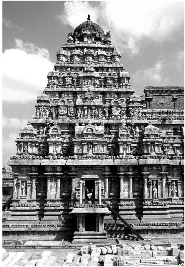
12. Airāvateśvara temple, Darasuram (Tamil Nadu), mid-twelfth century, a five-storey ( pañcatala ) vimāna . Unlike the equivalent temple in the Samarāṅgaṇa, here the kūṭa , pañjara , and śālā pavilions crowning the first and second tiers are two-storey ones ( ṣaḍvarga , ‘of six divisions’), i.e. equivalent to the entire śālā aedicule of Figure 6 (photo by Gerard Foekema).
