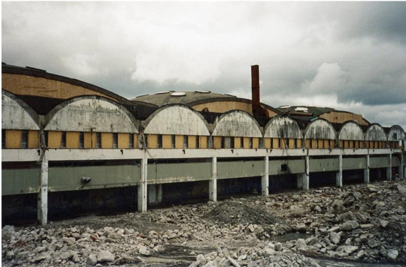
Rubber Factory, Brynmawr – 1951 Architects Co-Operative Partnership
