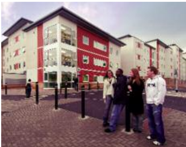
Talybont Court, the University's newest residence
