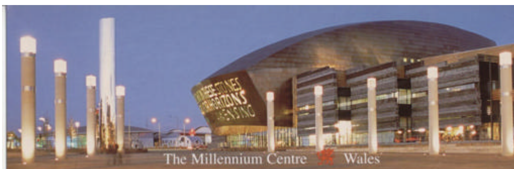
Figure 6: Wales Millenium Centre (building). © Neil Turner Photolibary.
