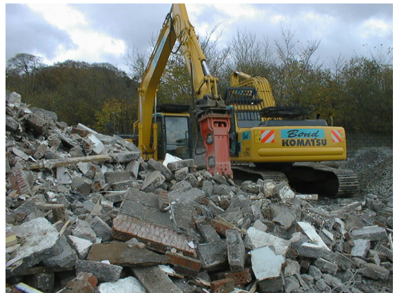
Figure 1 Crushing rubble for reuse
