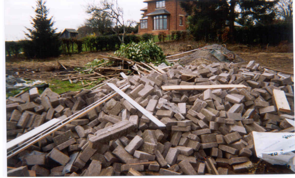
Figure 3 Reclaimed paving bricks for reuse
